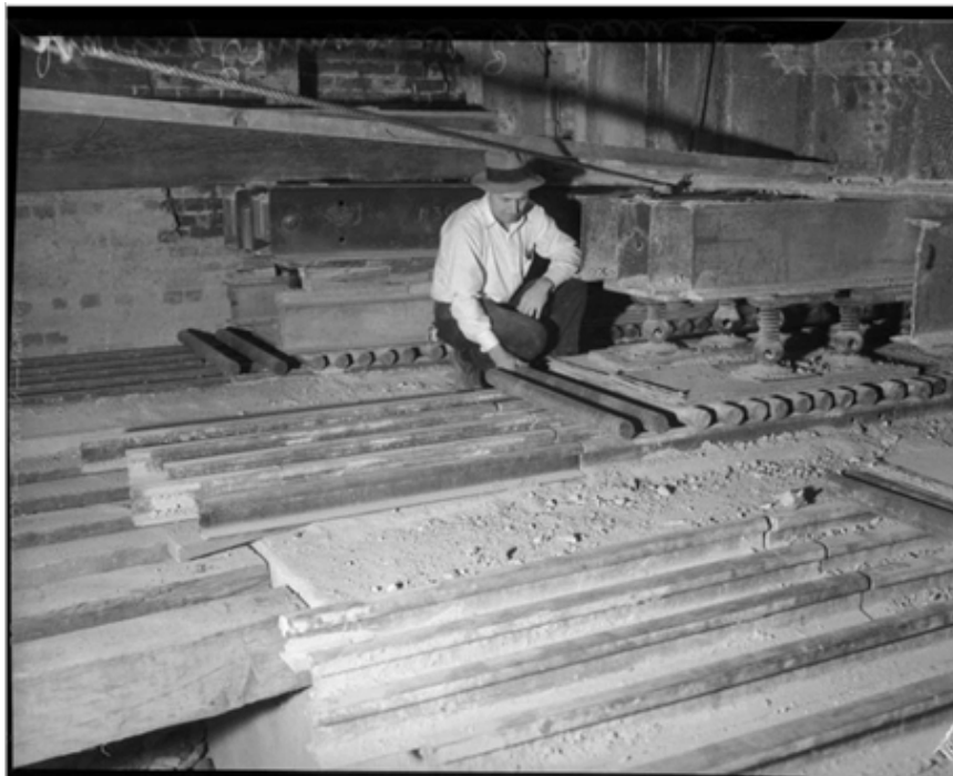
Figure 3. Building move, 1935, basement area as excavated to accomplish the move using steel rollers. Man is not identified in the archival record. Source: UCLA Online archives: http://digital2.library.ucla.edu/viewItem.do?ark=21198/zz00254xd6 .
