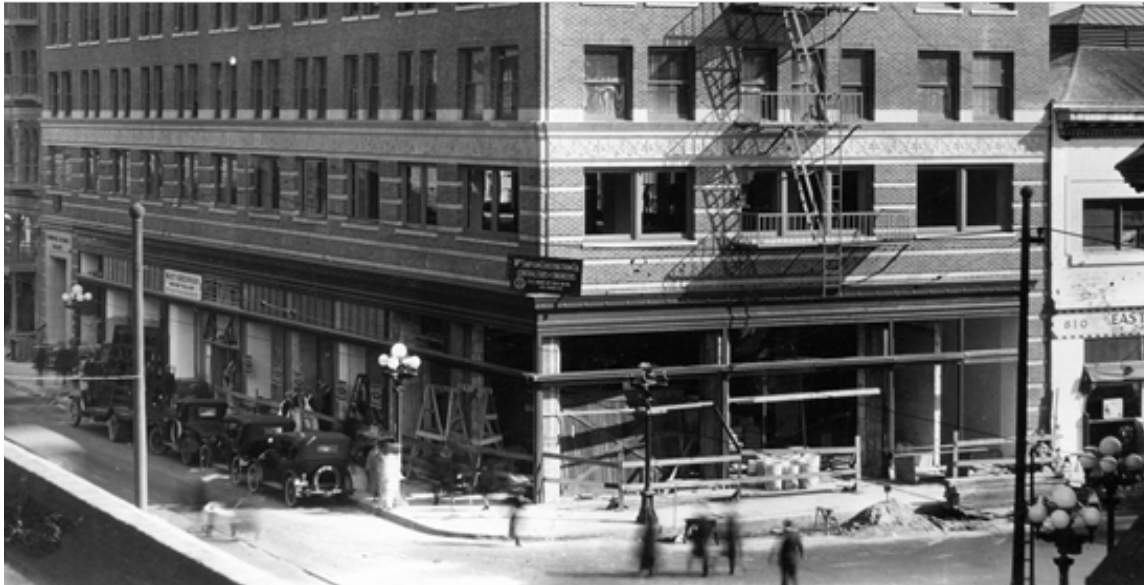
Figure 3. Building move, 1935, basement area as excavated to accomplish the move using steel rollers. Man is not identified in the archival record. Source: UCLA Online archives: http://digital2.library.ucla.edu/viewItem.do?ark=21198/zz00254xd6 .
