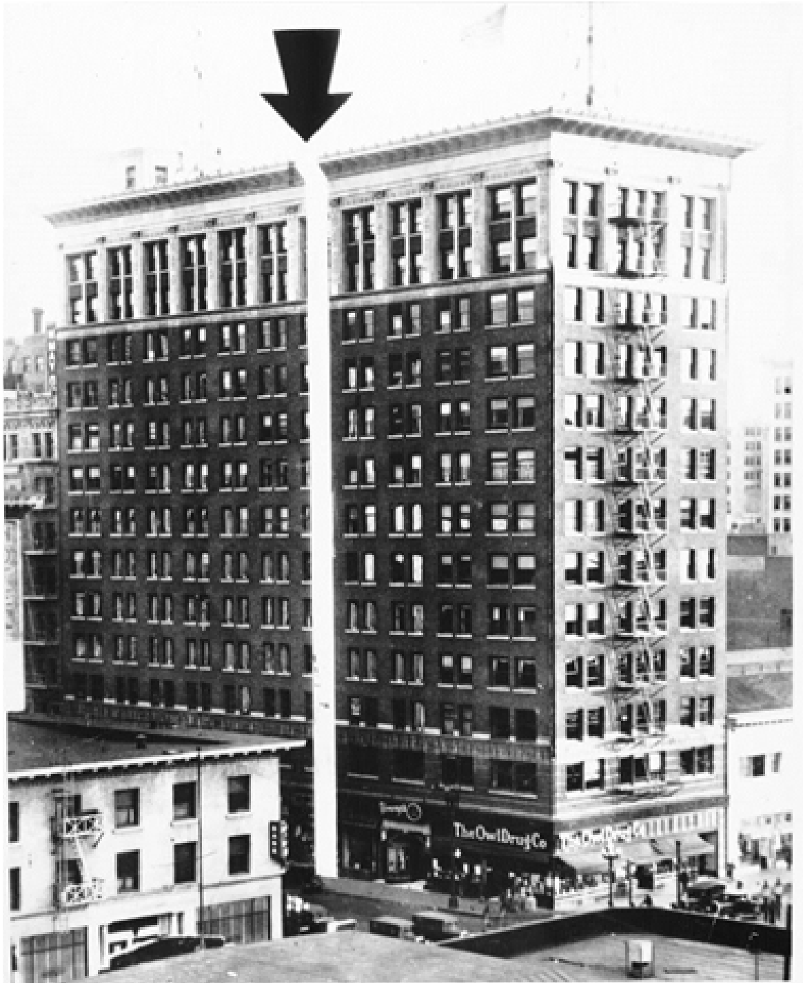
Figure 4. Image illustrates the location and scale of the cut made through the building to accommodate the move of the west portion in 1935. Los Angeles Examiner , USC Special Collection (EXM-P-S-LOS-ANG-CIT-BUI-055)
